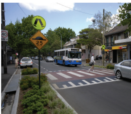
Raised pedestrian crossing
