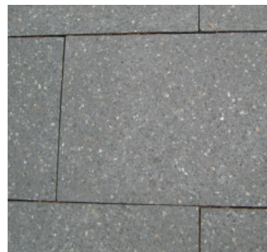
Concrete unit paving
