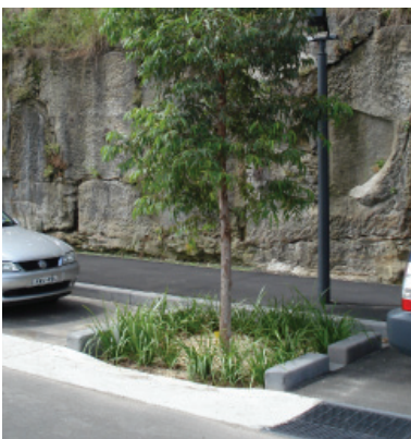
Dish drains and open pit raingardens
