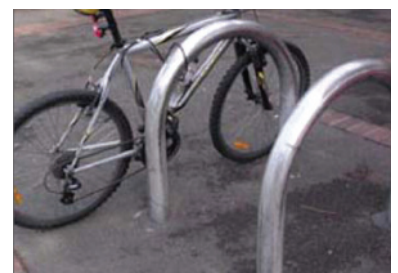
U-racks bicycle storage
